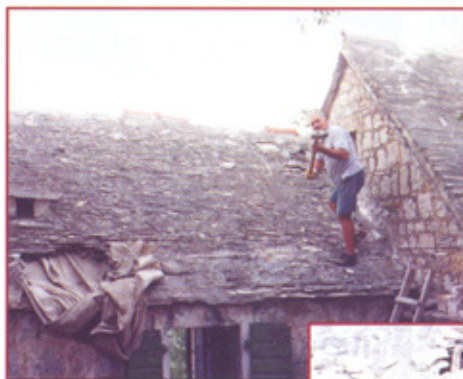
Figures 6a and 6b: Beginning of work; taking stone tiles down from the roof.
