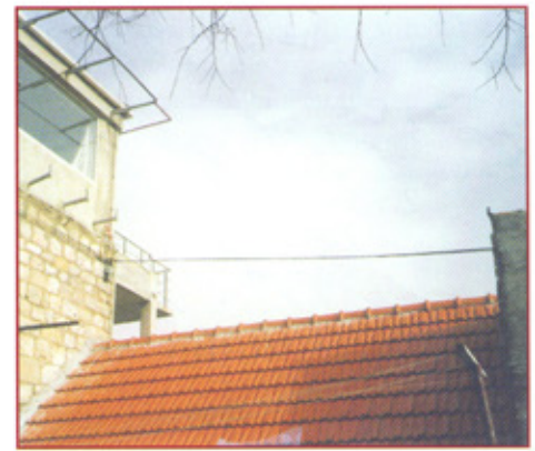
Figure 14: The roof repair is finally done properly.
