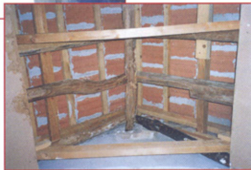
Figures 10a and 10b: Corrective attempts from inside; attic boards and joists were later removed.
