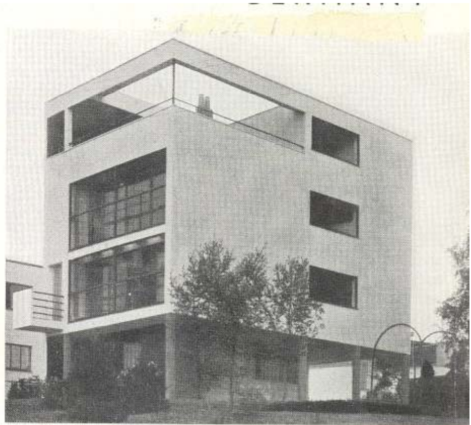
THE SINGLE HOUSE. Posts are spaced regularly, without regard to interior arrangements, so that planning is free, divisions on one floor being independent of divisions on another; posts rise directly from the ground, raising the living floor above ground dampness. These vertical posts and horizontal floors leave spaces in the façade through which light and air may penetrate freely.
